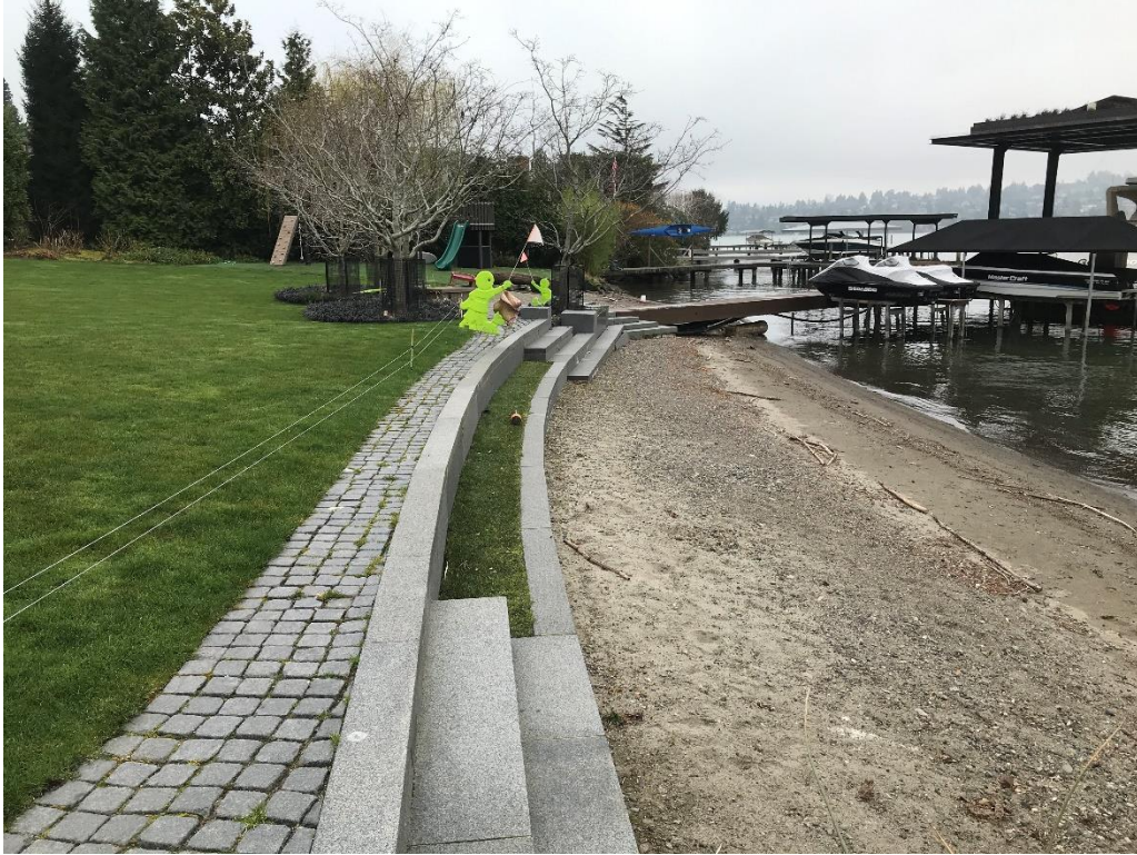
Photo 7. View of shoreline from north property line looking south.
