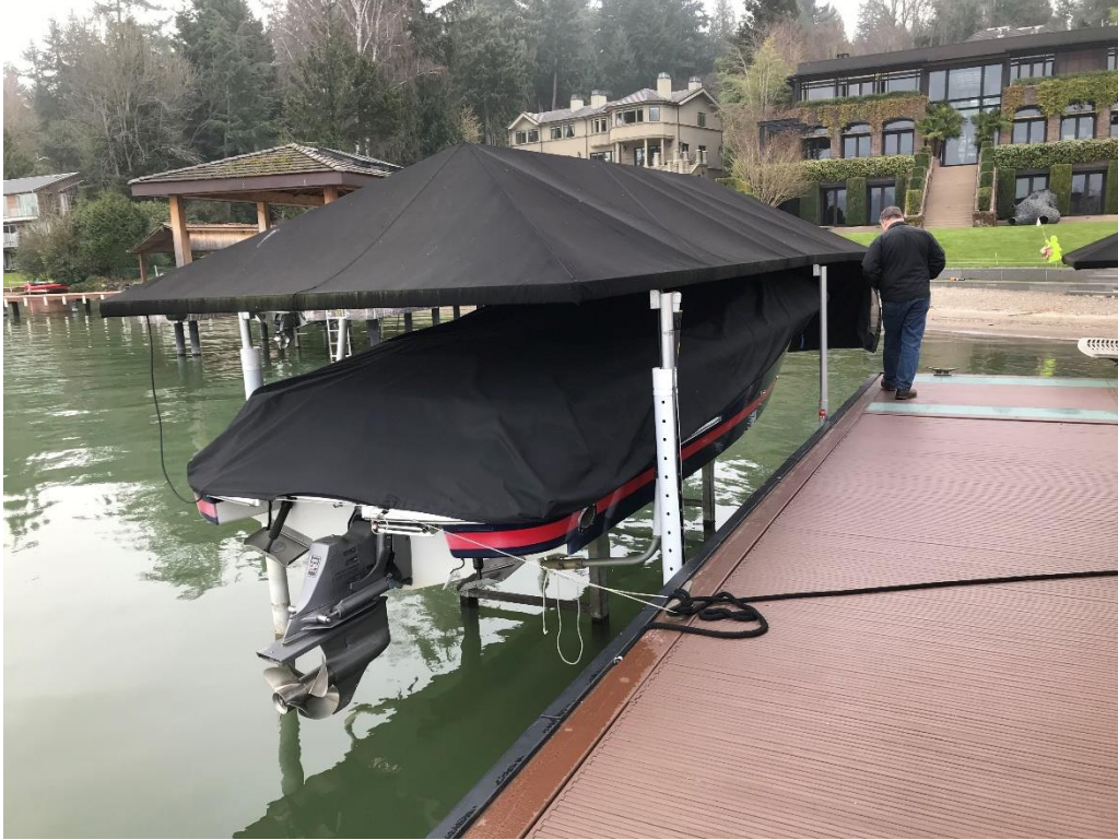
Photo 3. View of pier from northwest corner looking east.
