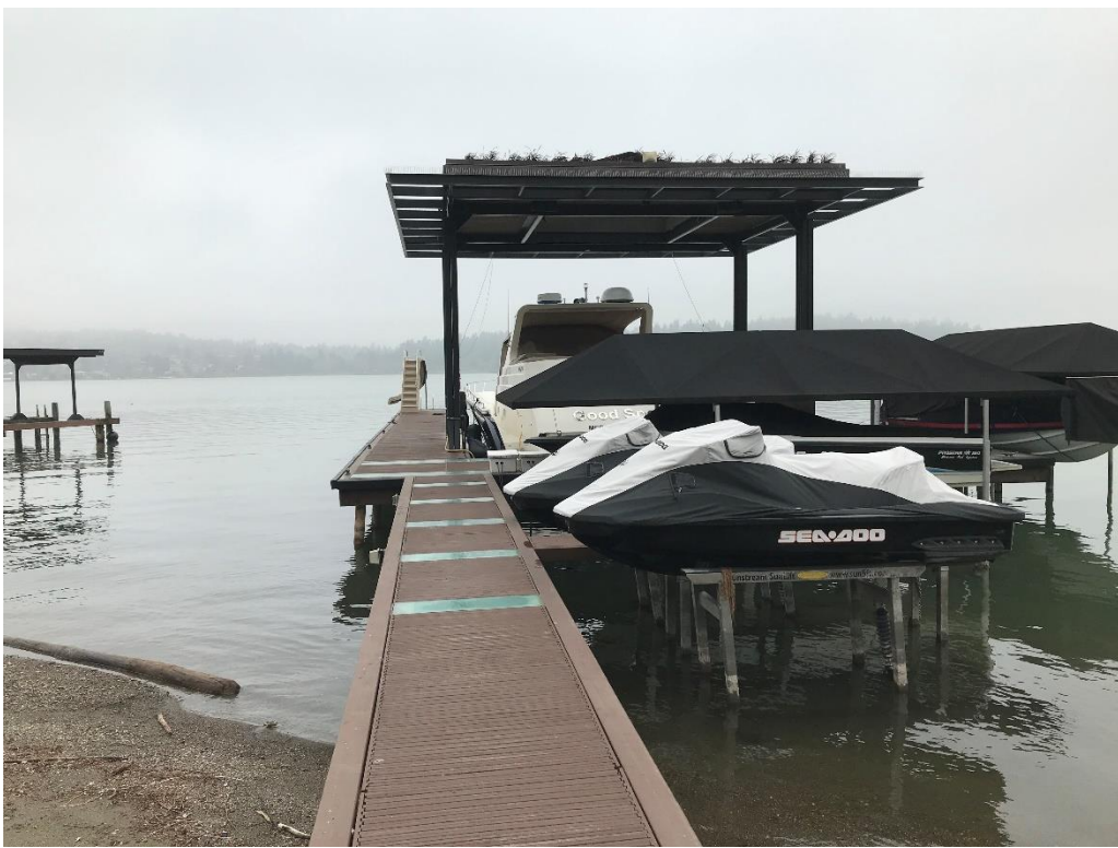
Photo 1. View of north pier from shore looking west.
