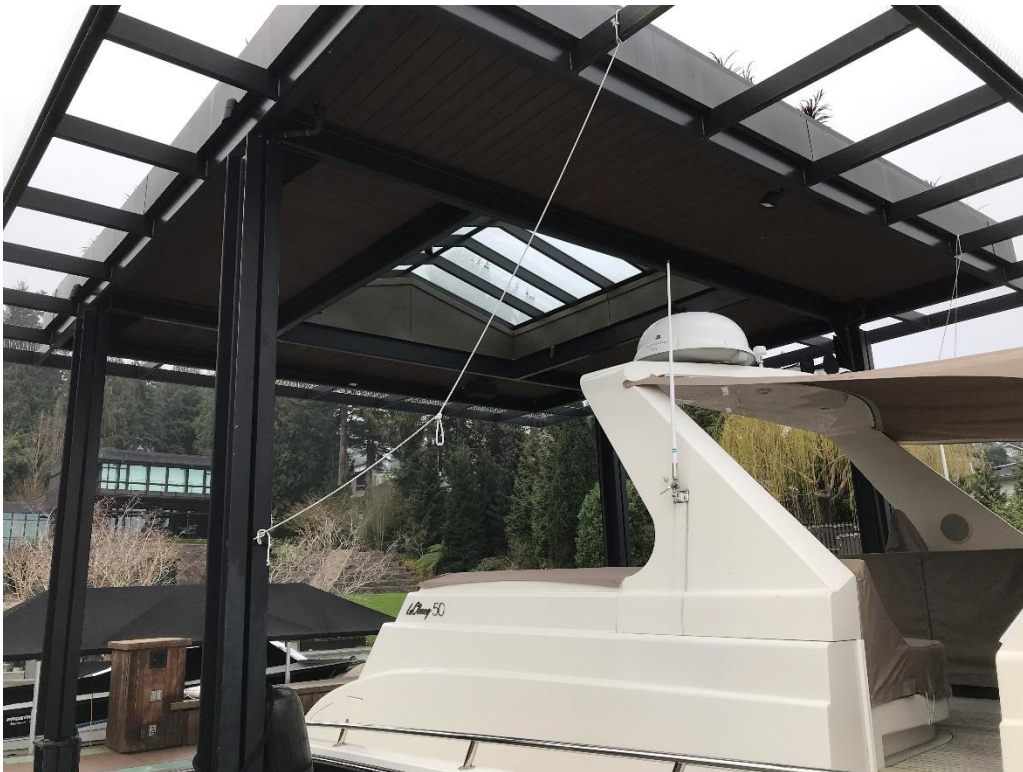
Photo 4. View of moorage cover from northwest corner.
