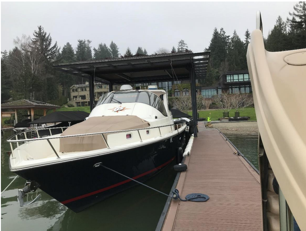
Photo 2. View of pier from southwest corner looking east.
